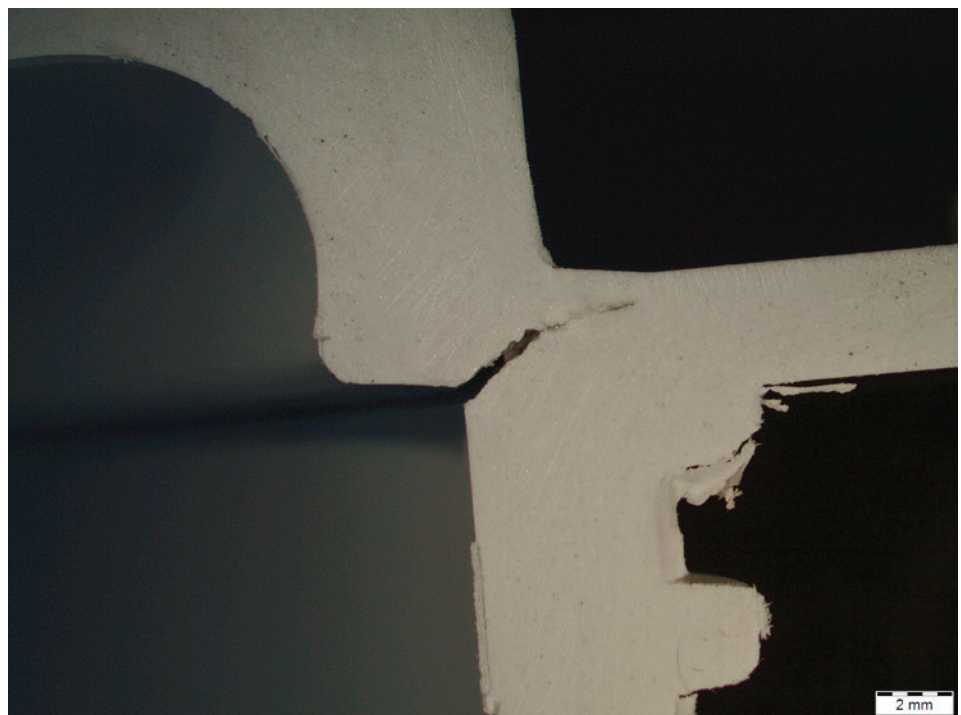
Figure 1—A plastic water filter manifold that has failed at an abrupt transition in the part geometry.
